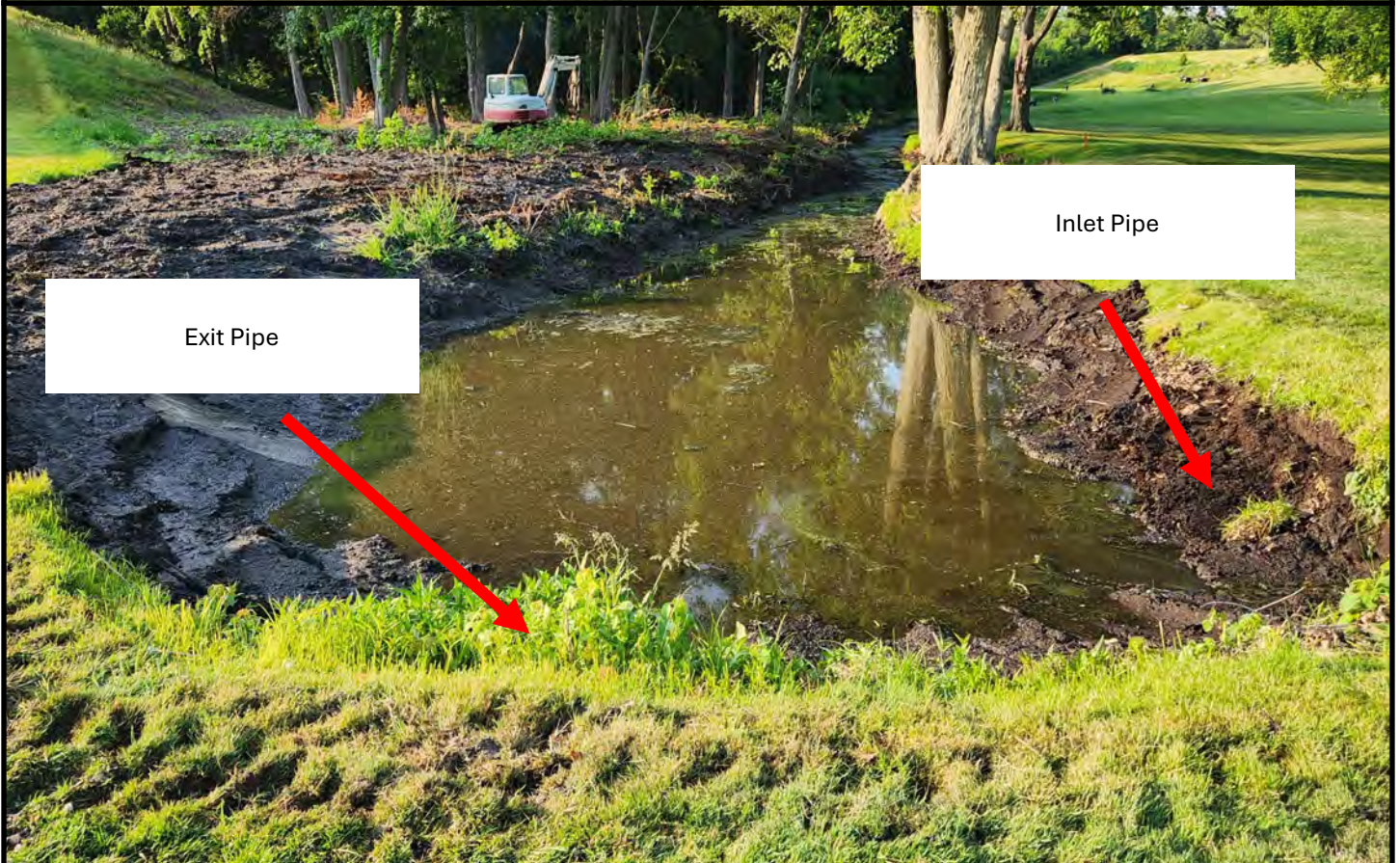
The bottom photo is the collection area where water from the clubhouse, #1, 2, 3, 8, and 9 enters through a pipe. The water then exits through a different pipe into the marsh right side of #7
