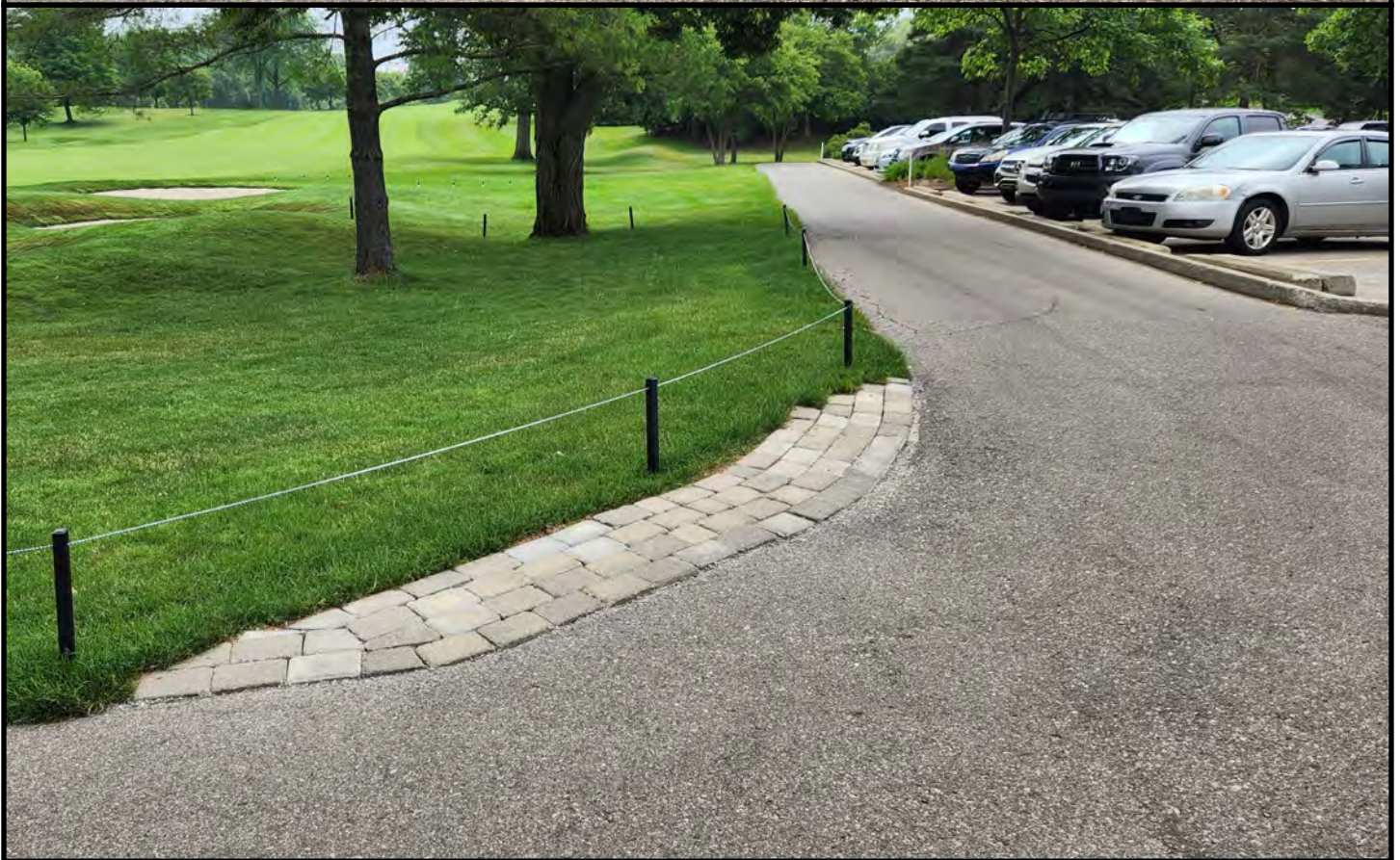
Pavers and sod installed to the left side of #9 green.
