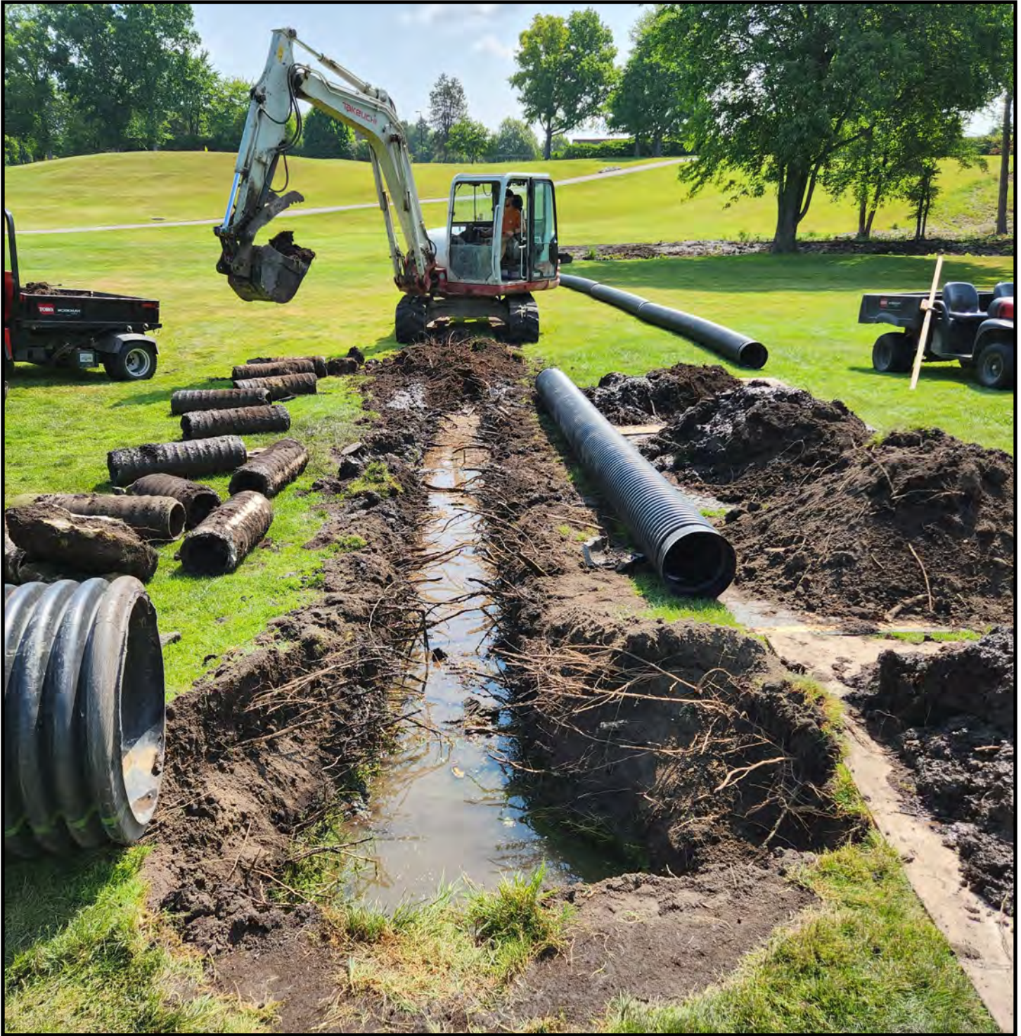
The excavator installing the new corrugated pipe to the right of the photo. The old concrete pipe is in sections on the left side of the photo. The new pipe is 2" bigger in diameter which will allow for slightly more water flow through this portion of the system.
