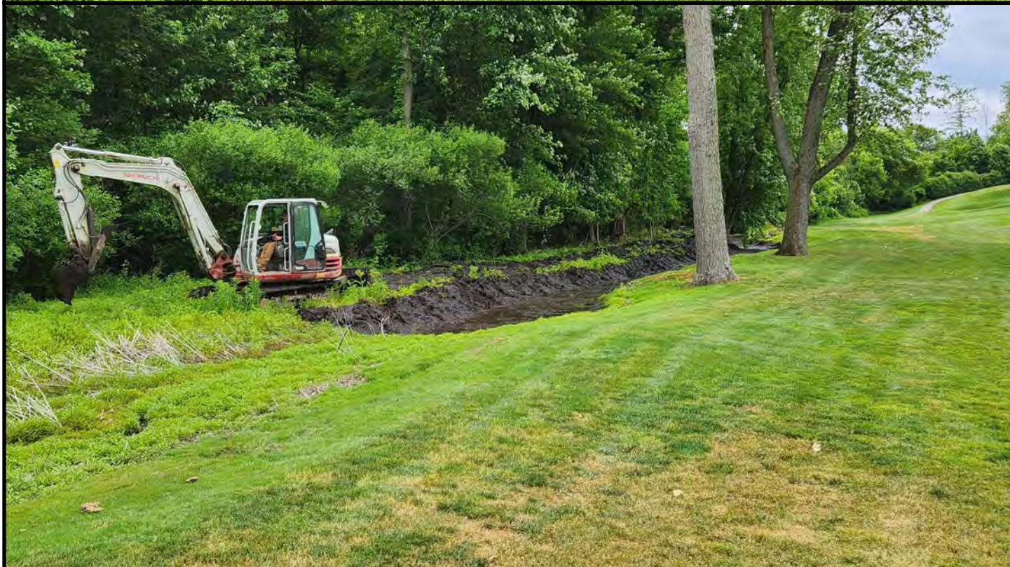
Excavator dredging the ditch left of #8. We are happy with the increased volume of water this ditch can hold after rain events.
