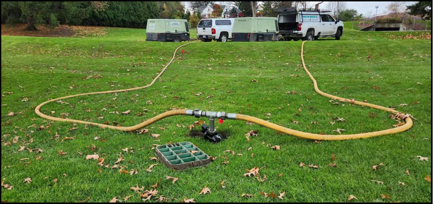
2 air compressors are hooked into the piping to provide enough pressure and volume to clear the irrigation system of water
